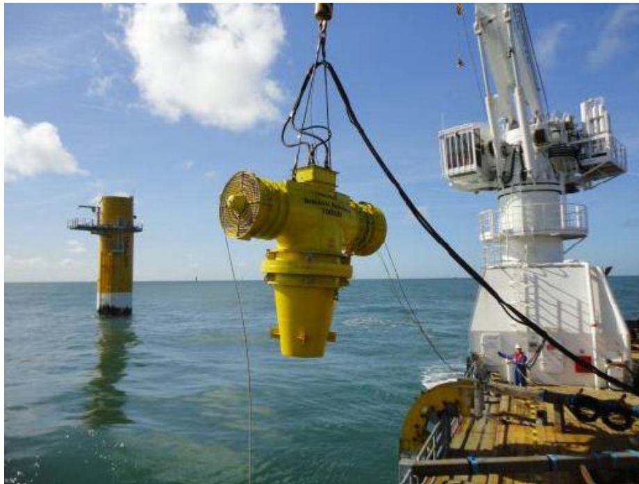
Figure 5: Mass Flow Excavator Tool
